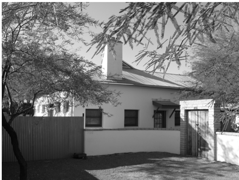
Photograph 22. 950 S. 8th Ave.; view west-northwest.
