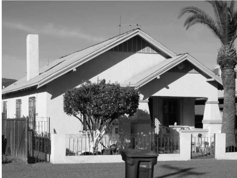
Photograph 7. 930 S. 8th Ave.; view west-northwest.
