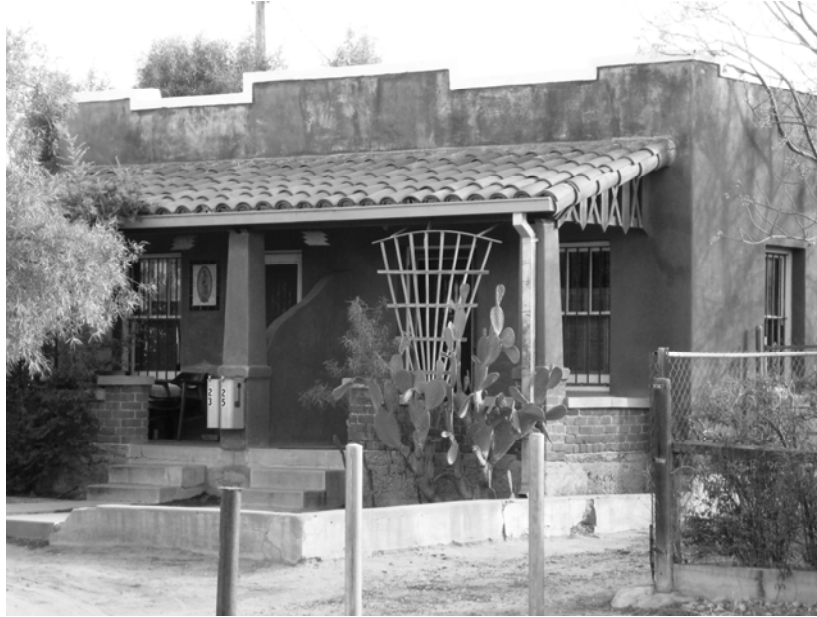
Photograph 23. 23-25 W. 19th St.; view south-southeast.
