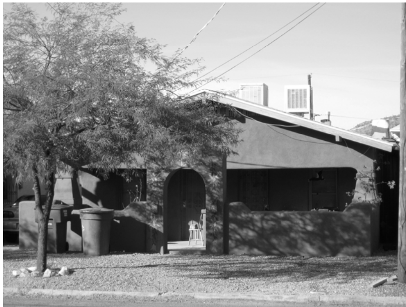
Photograph 6. 928 S. 8th Ave.; view west-southwest.
