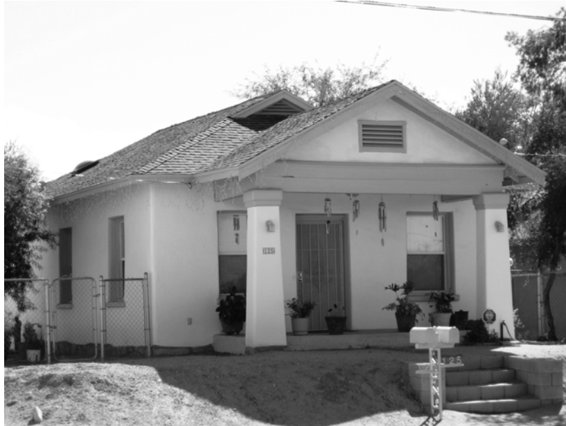
Photograph 5. 125 W. 19th St.; view south-southwest.
