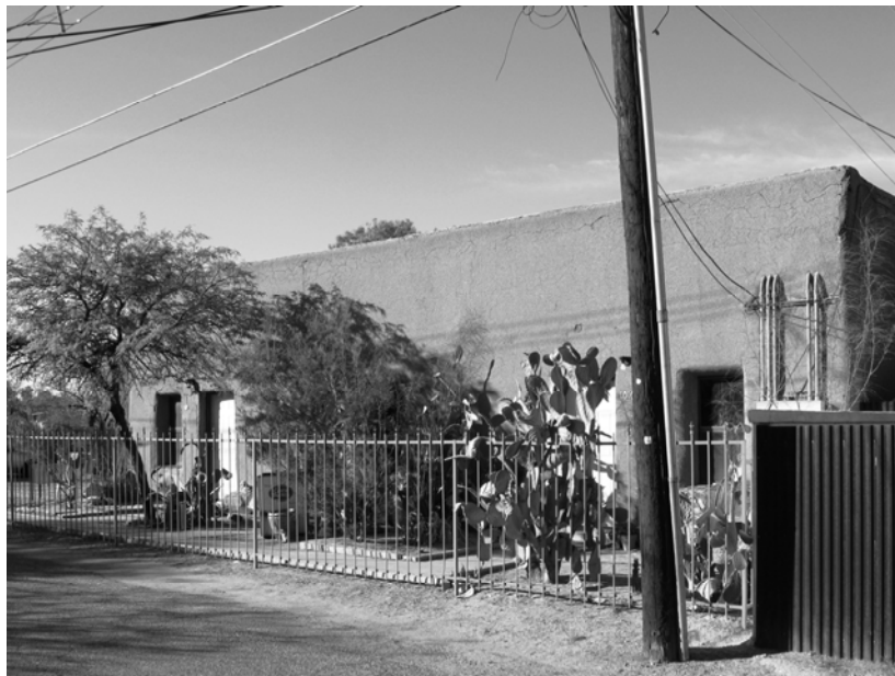
Photograph 24. 1010-1014 S. Rubio Ave.; view west-southwest.
