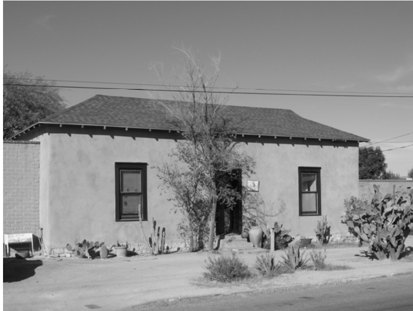
Photograph 25. 904 S. 8th Ave.; view west-northwest.
