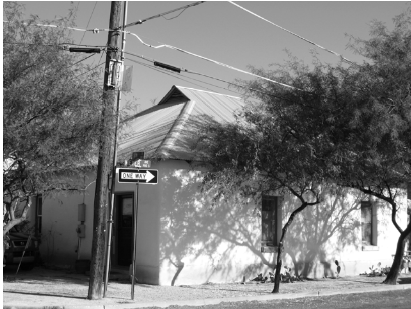
Photograph 11. 901 S. Meyer Ave.; view east-southeast.
