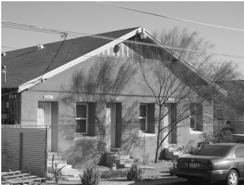
Photograph 2. 1015-1019 S. Meyer Ave.; view east-southeast.
