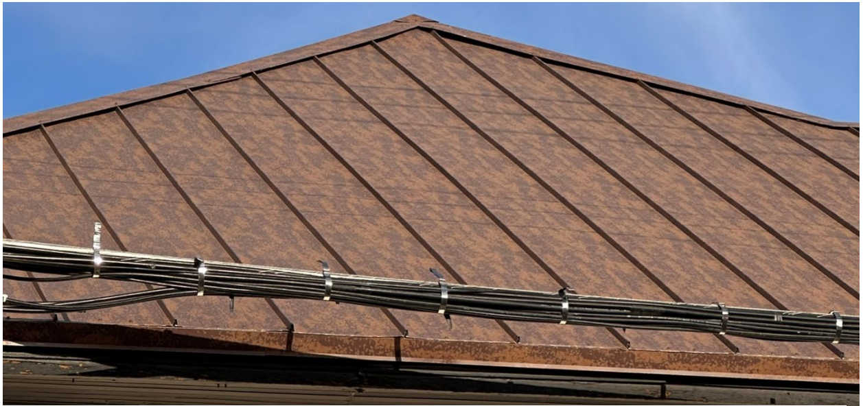
Close-up of standing seam metal roof system, March 2025
