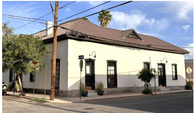
Current Metal Panel Roof, March 2025
