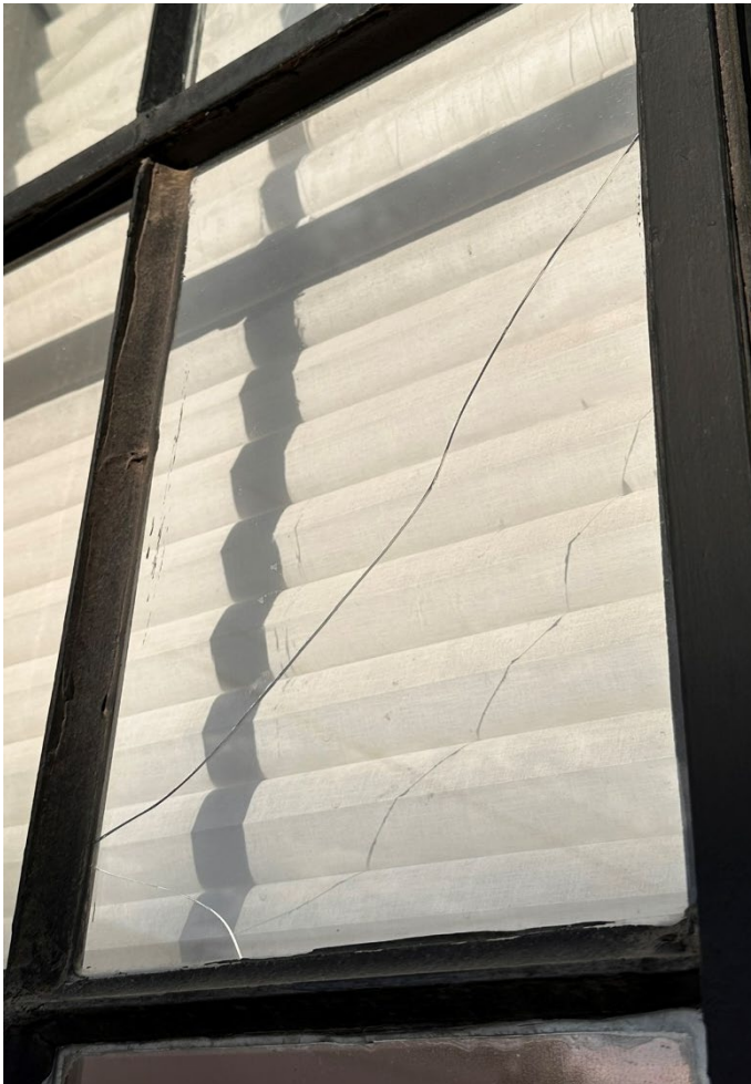
Broken single-pane plate glass windows, March 2025
