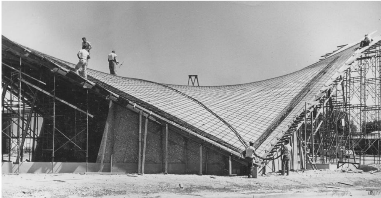
Catalina Baptist Church, under construction c. 1959.
