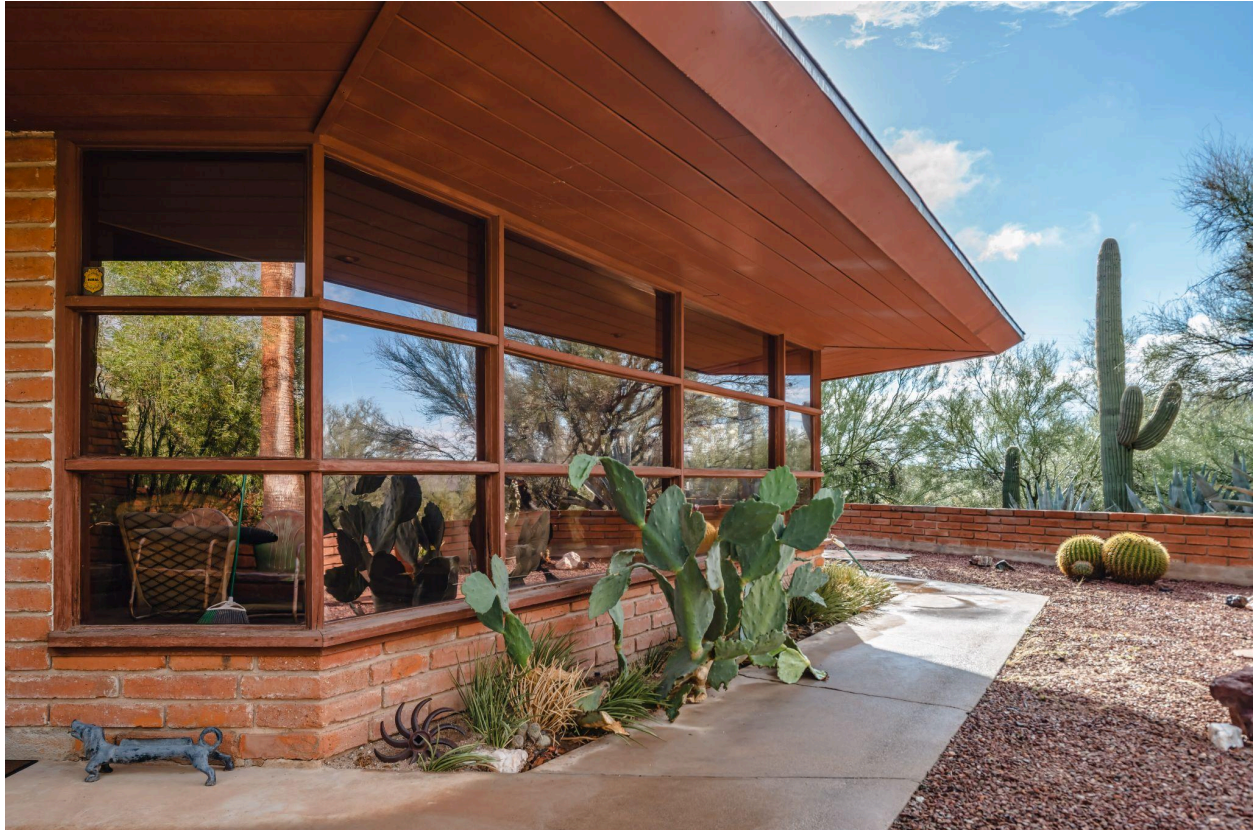
Charles Cox House, South Elevation, Photo by GMVargas 2023
