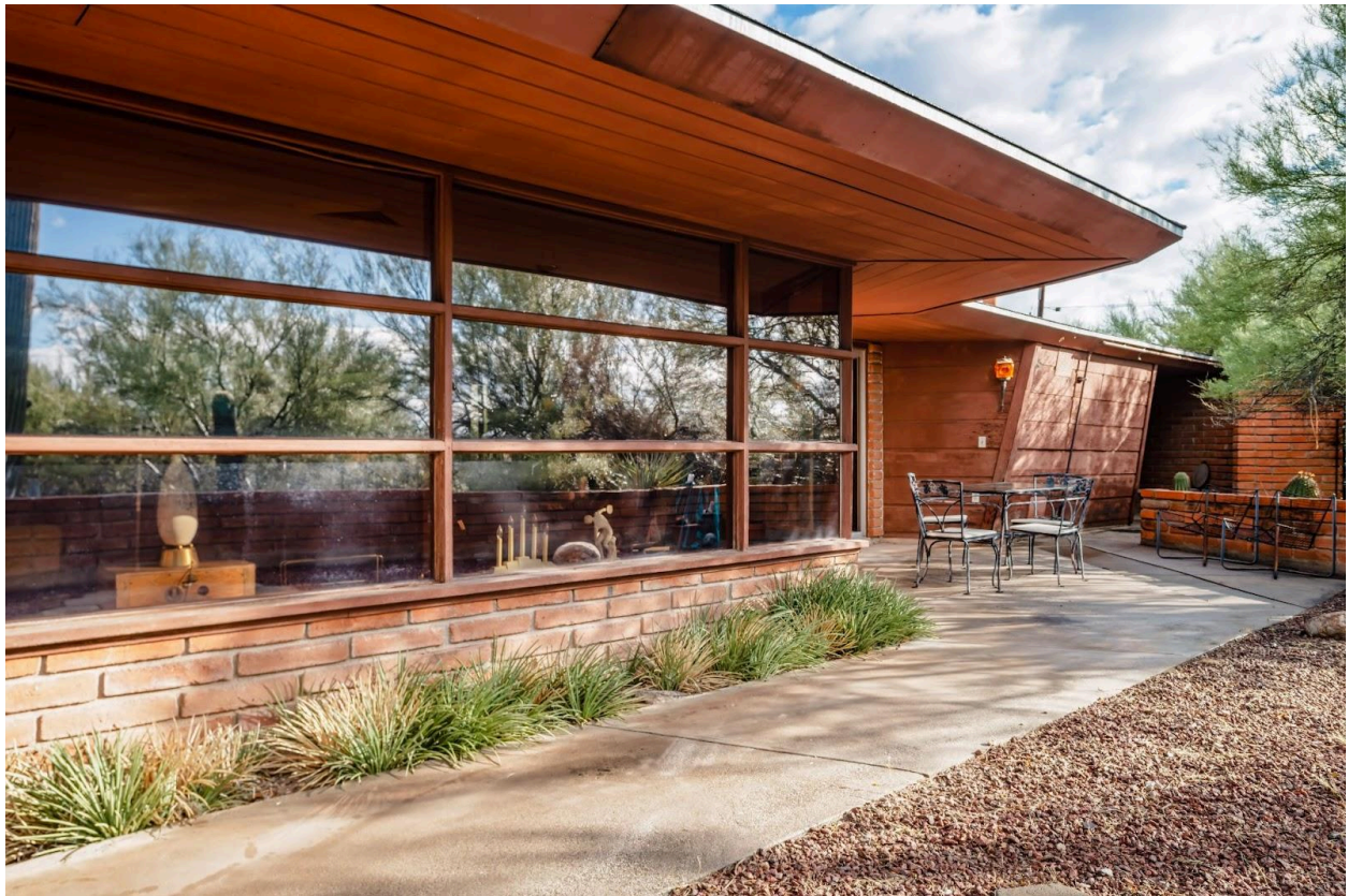
Charles Cox House, South elevation, living room window.
