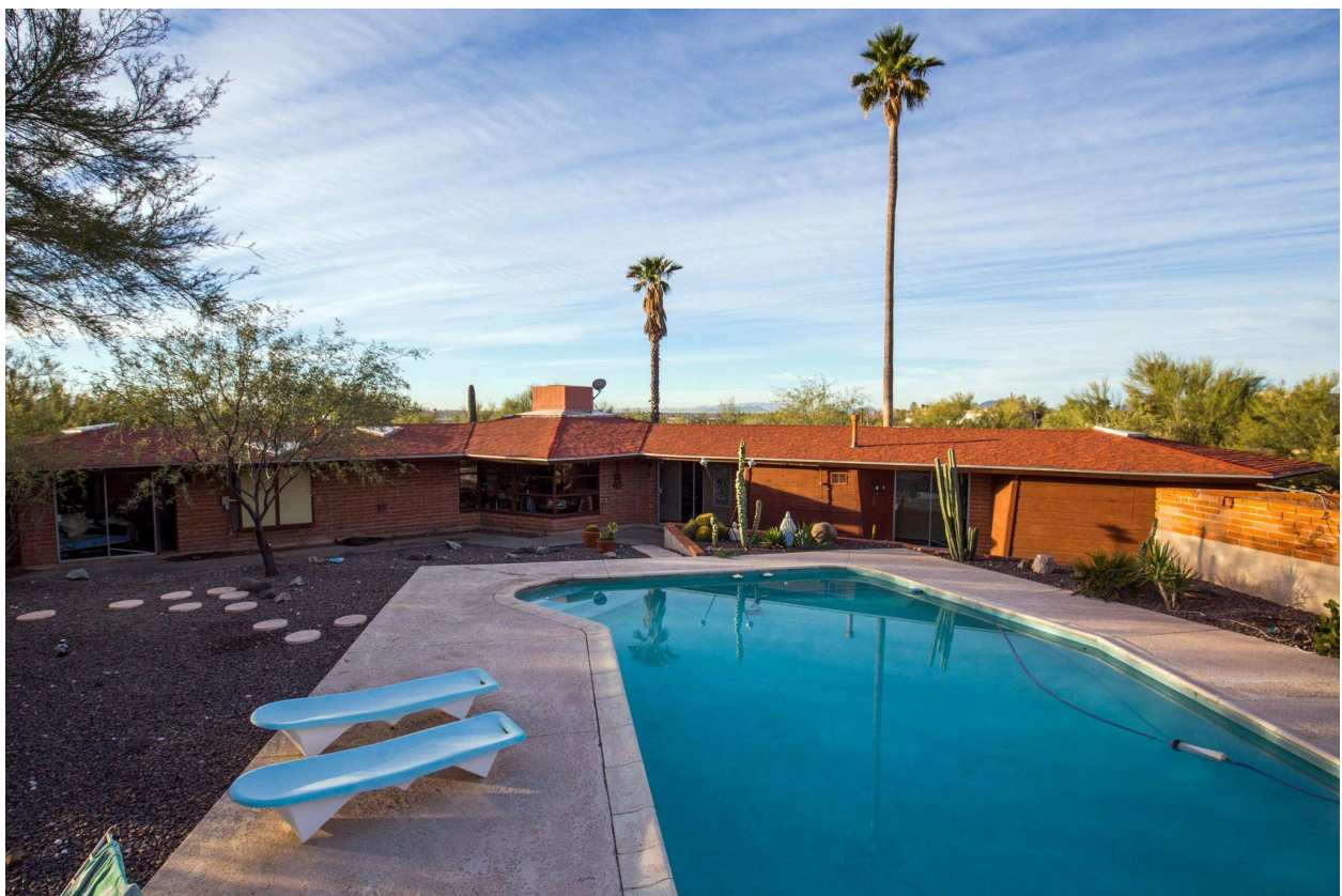
Charles Cox House, North Elevation, Photo by Reed, 2023
