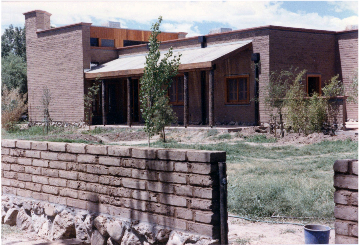
Home After Construction, west elevation, Russell-Randolph Photo Collection, c. 1983
