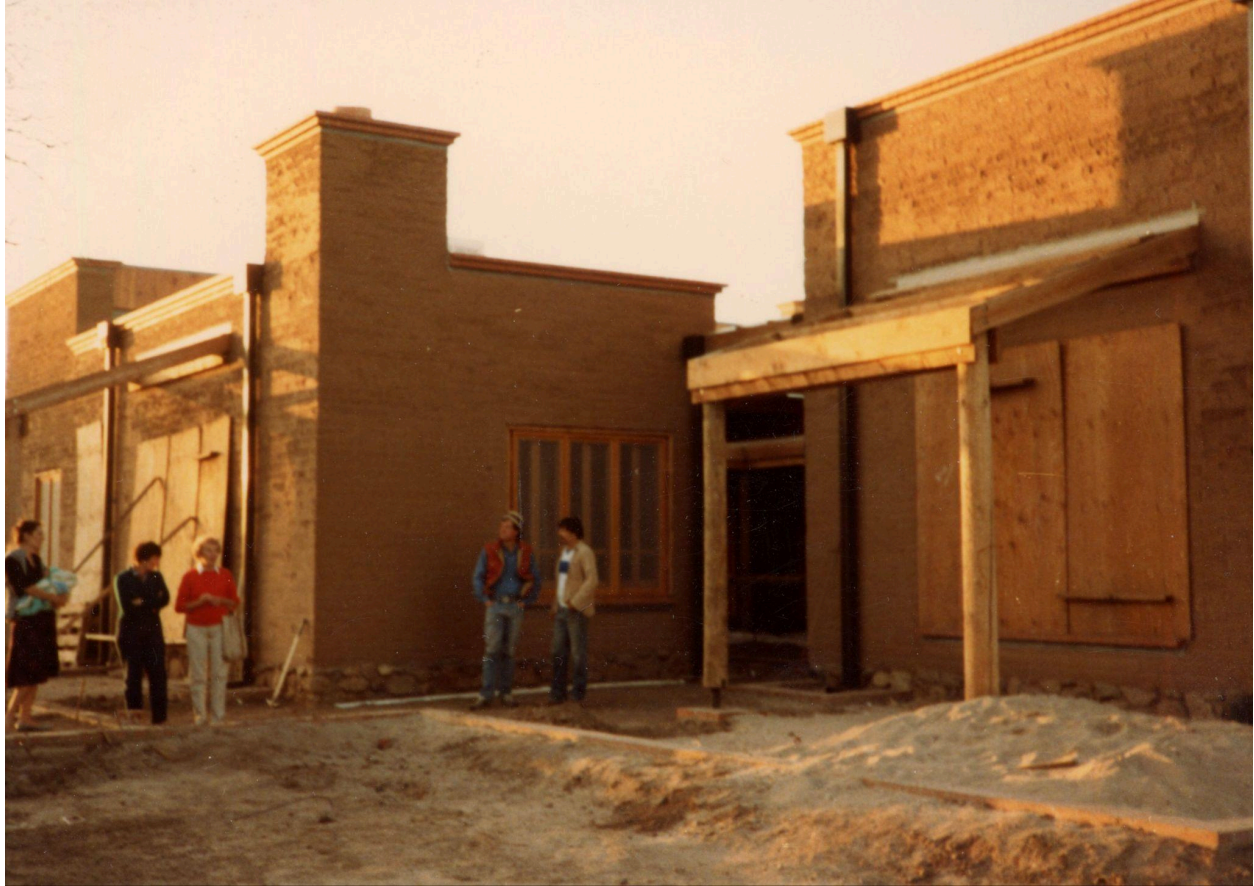
Home Under Construction, Russell-Randolph Photo Collection, c. 1983
