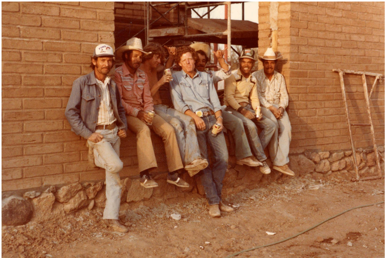
Home Under Construction, Construction Crew, Russell–Randolph Photo Collection, c. 1983
