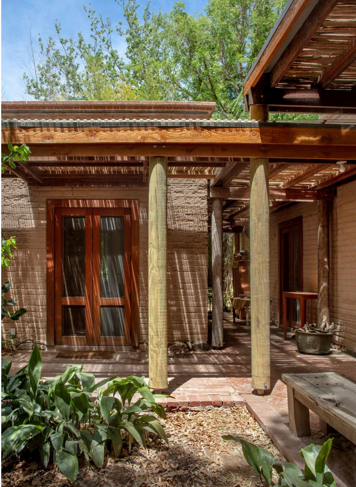
Courtyard looking north, Bill Timmerman, 2019
