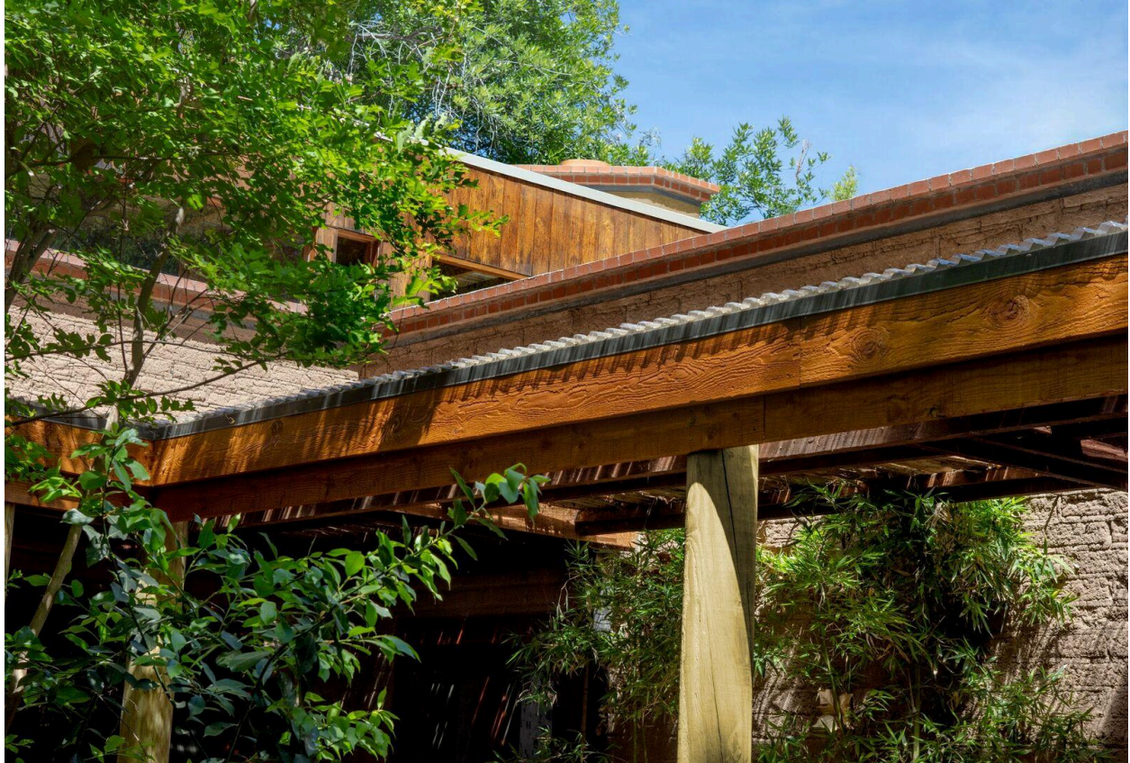
Exterior covered walkway detail, Bill Timmerman, 2019
