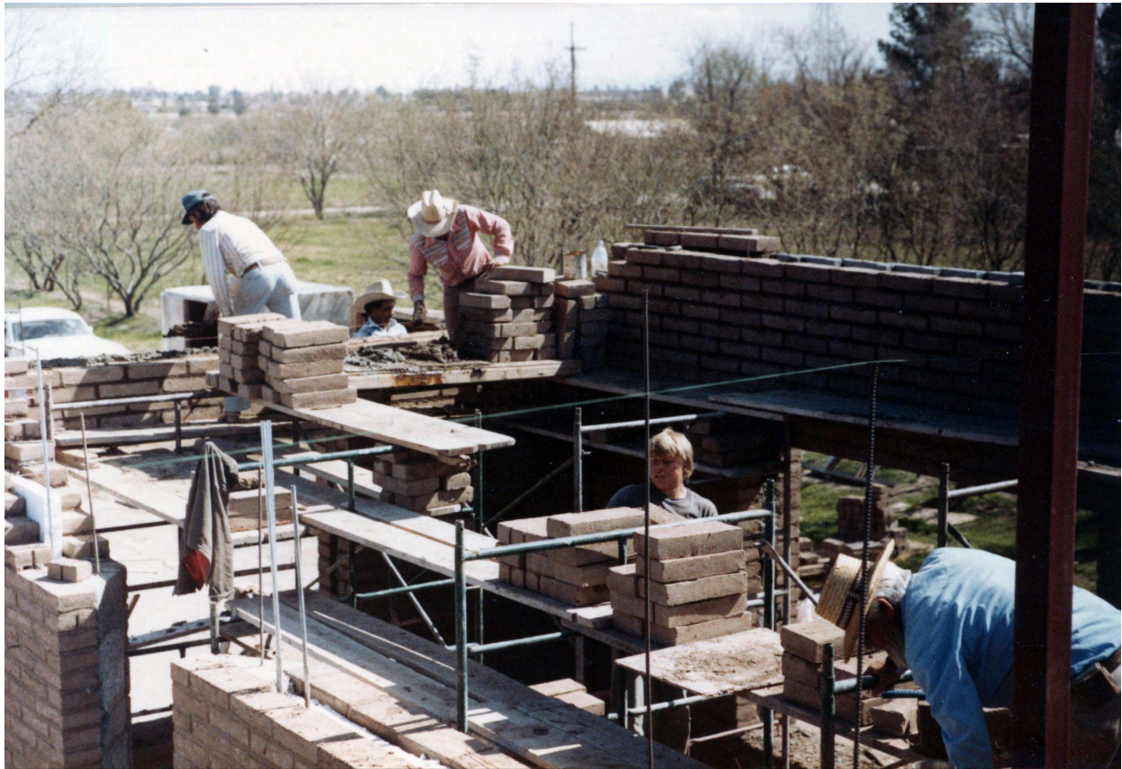
Home Under Construction, Russell-Randolph Photo Collection, c. 1982
