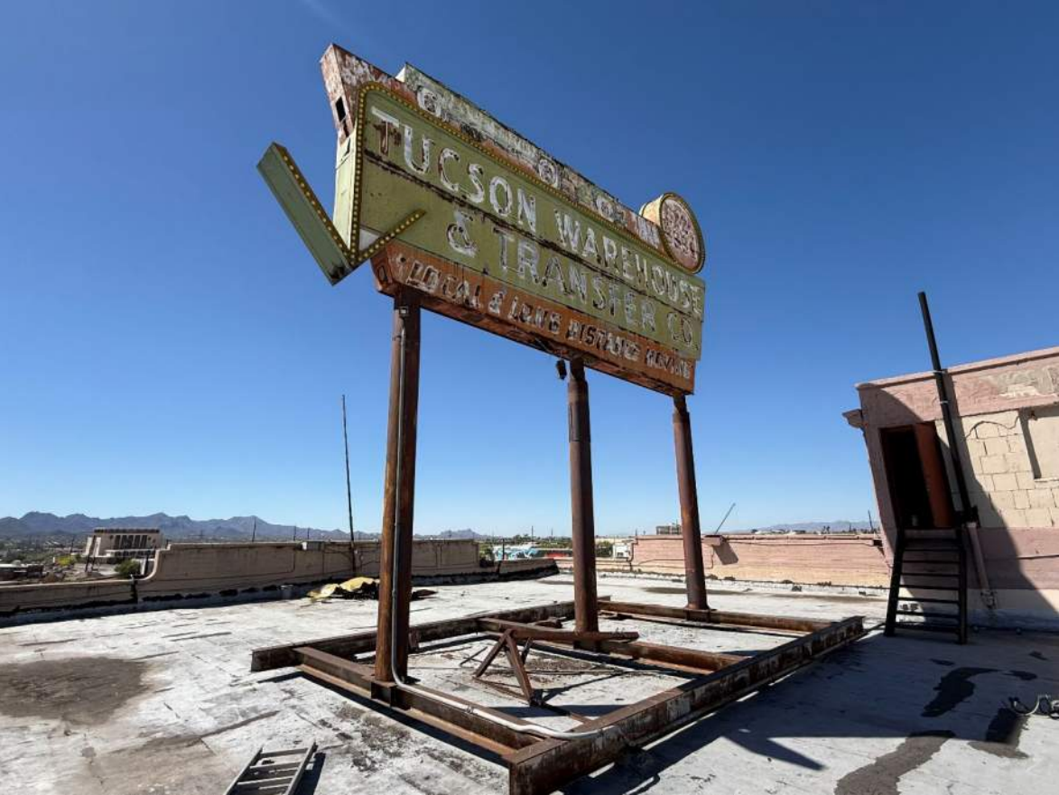
VIEW FACING NORTHWEST
