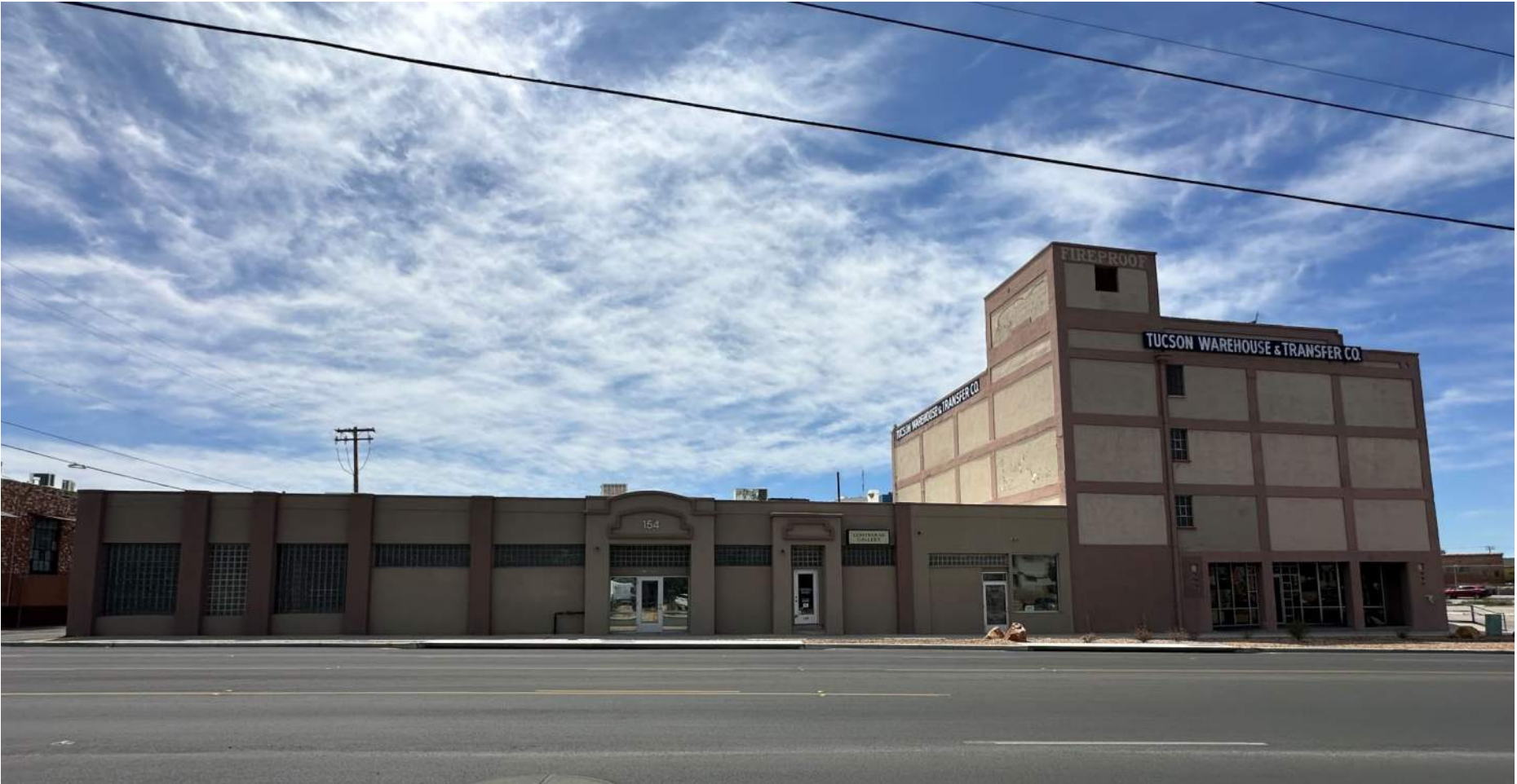
NORTH ELEVATION FROM E. 6TH ST.
