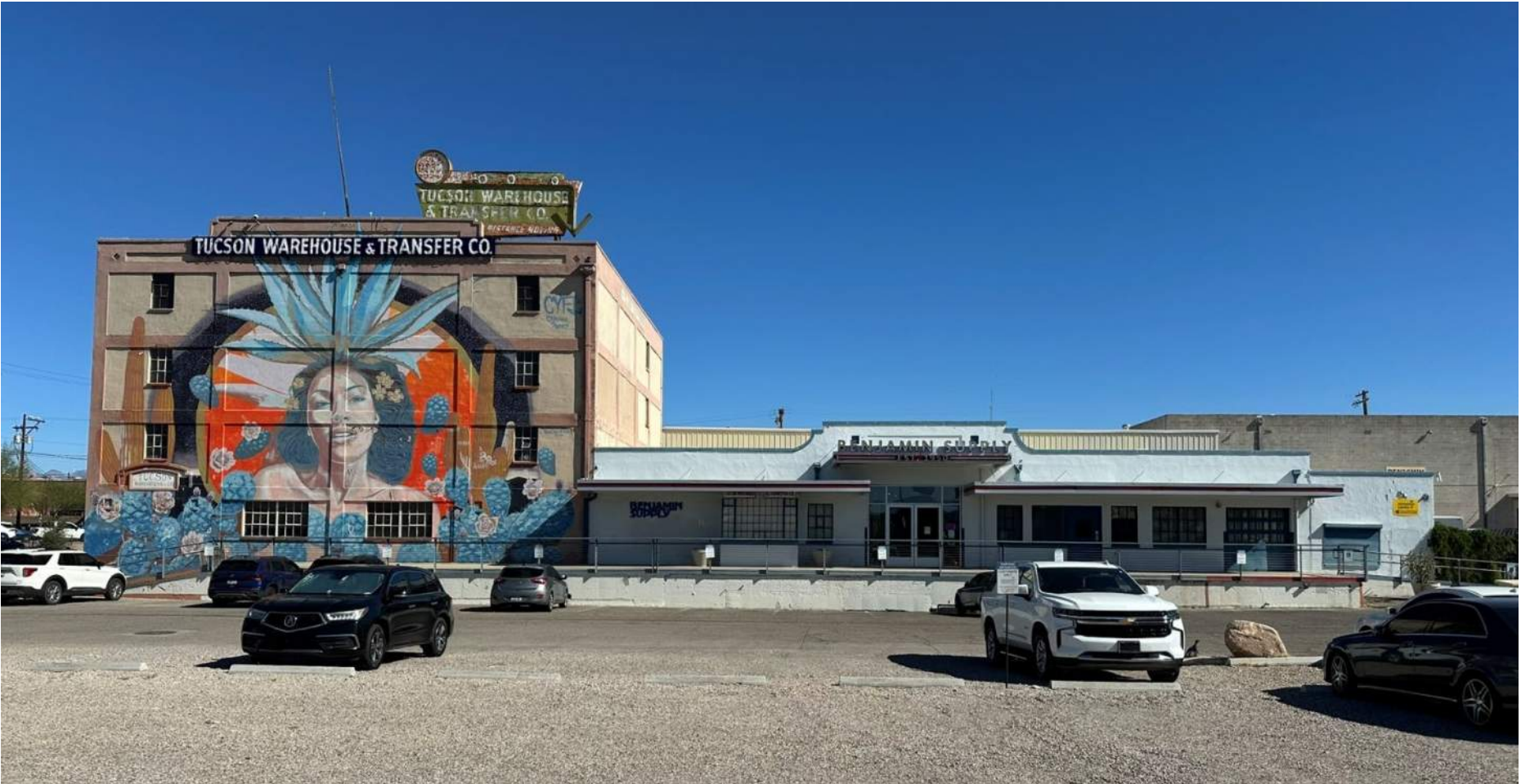
WEST ELEVATION FROM MACLOVIO BARRAZA PARKWAY
