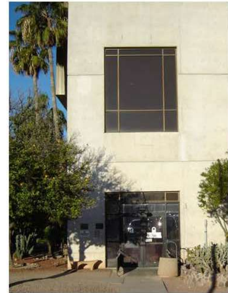
CAST-IN-PLACE CONCRETE, ALUMINUM STOREFRONT
