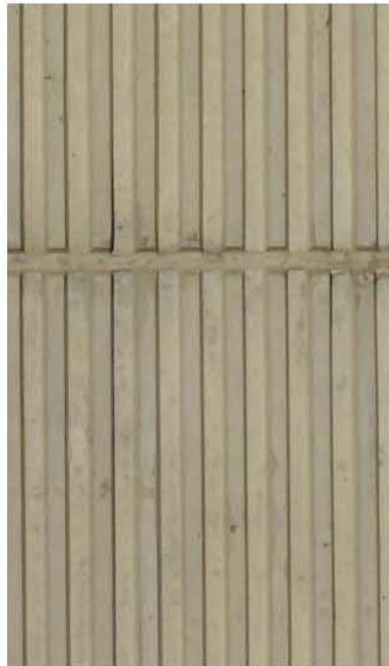
CAST-IN-PLACE CONCRETE RIBBED FORM TEXTURE
