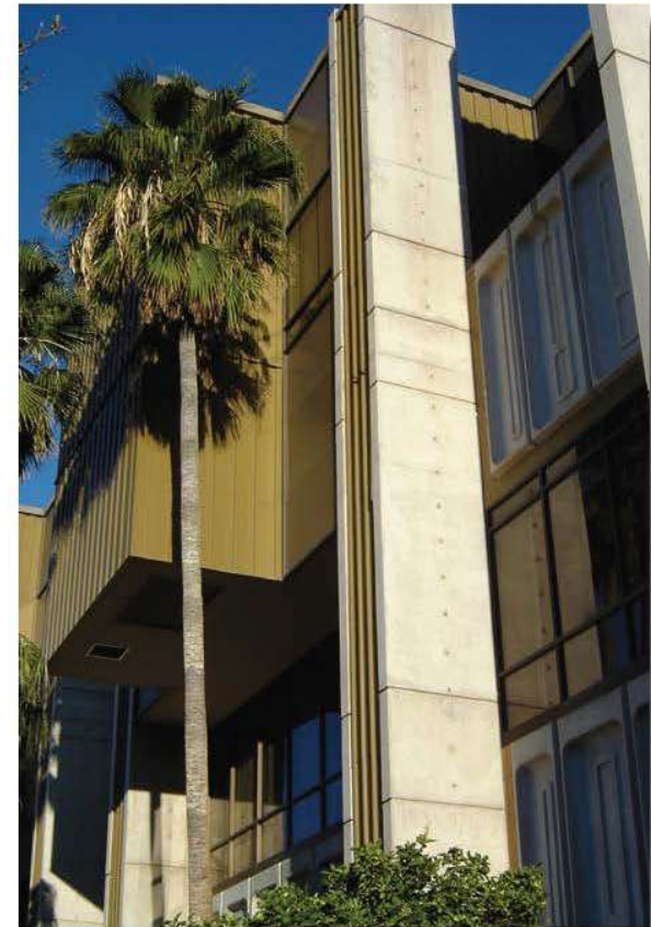
CAST-IN-PLACE CONCRETE, PRE-FINISHED METAL PANELS, ALUMINUM STOREFRONT
