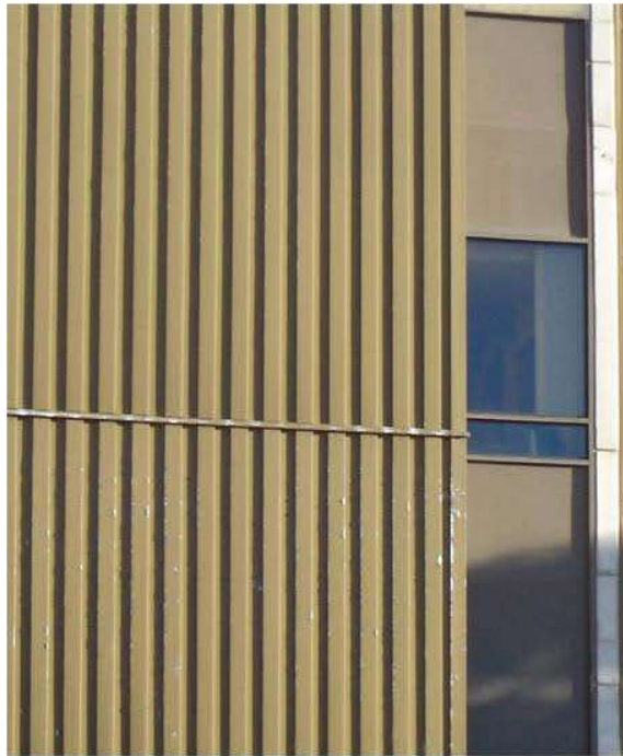
PRE-FINISHED METAL PANELS, ALUMINUM STOREFRONT
